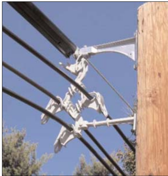
Figure 1-1: Hendrix Covered Conductor System
